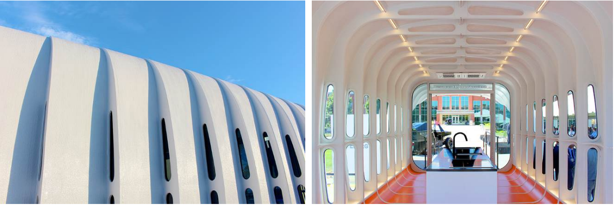
Figure 3 Left: Joined rings from exterior; Right: Joined rings from interior.
