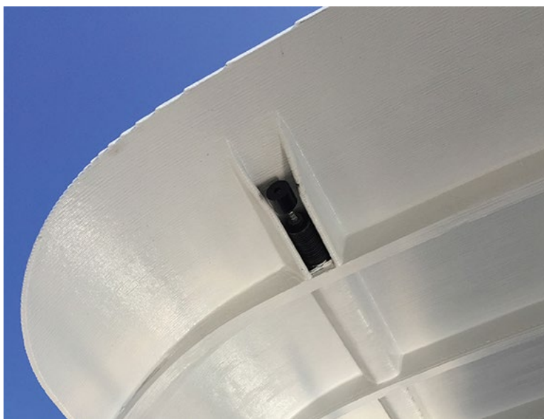
Fig. (9): Left: Detail of the pre-tensioned rod sleeve and light fixture socket; Right: 3D printed canopy with incorporated rod sleeve and disk spring pocket.
