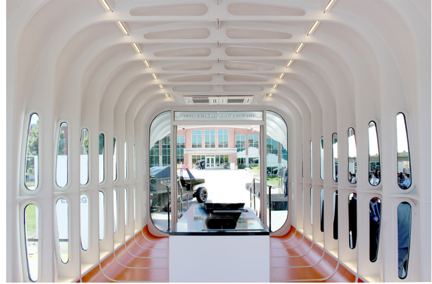
Fig. 6 Daylighting in the AMIE structure
