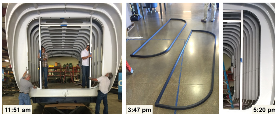
Fig. 14 Replacement of over-sized end wall frames using 3D-printed sections
