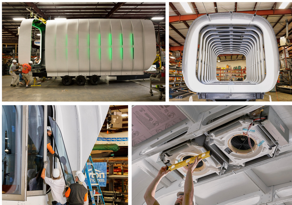
Fig. 8 Assembly of the AMIE structure
